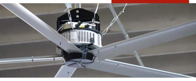
HVLS fans stand for High Volume Low-Speed fans. They have greater than 2.1 meters diameter and this ensures a large volume of air displacement. A single HVLS fan can replace multiple normal wall fans and still give a better performance. It saves about 80% cost of operating within 6 months of installation.
